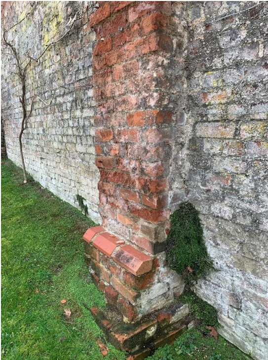
A buttress supporting a tall boundary wall.
