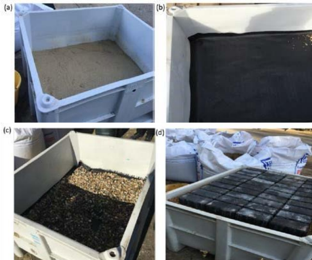
Figure 4. (a) Design one with Subgrade layer (sand) levelled, (b) Geotextile membrane fixed in place and (c) Sub-base layer filling and (d) 123mm of laying recycled coarse material placed, alongside 40 permeable blocks on Permeable Pavement System at the University of Greenwich, Medway Campus
