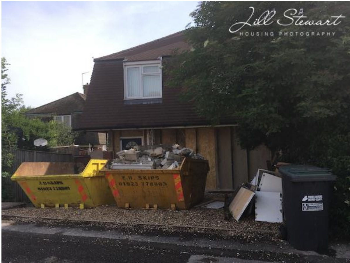
Cornish house under renovation, photographed 2022 (see also Post 2 next week)
