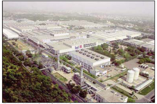
The original Maruti Suzuki facility at Gurgaon now comprises three plants with capacity for 700,000 units per annum.
