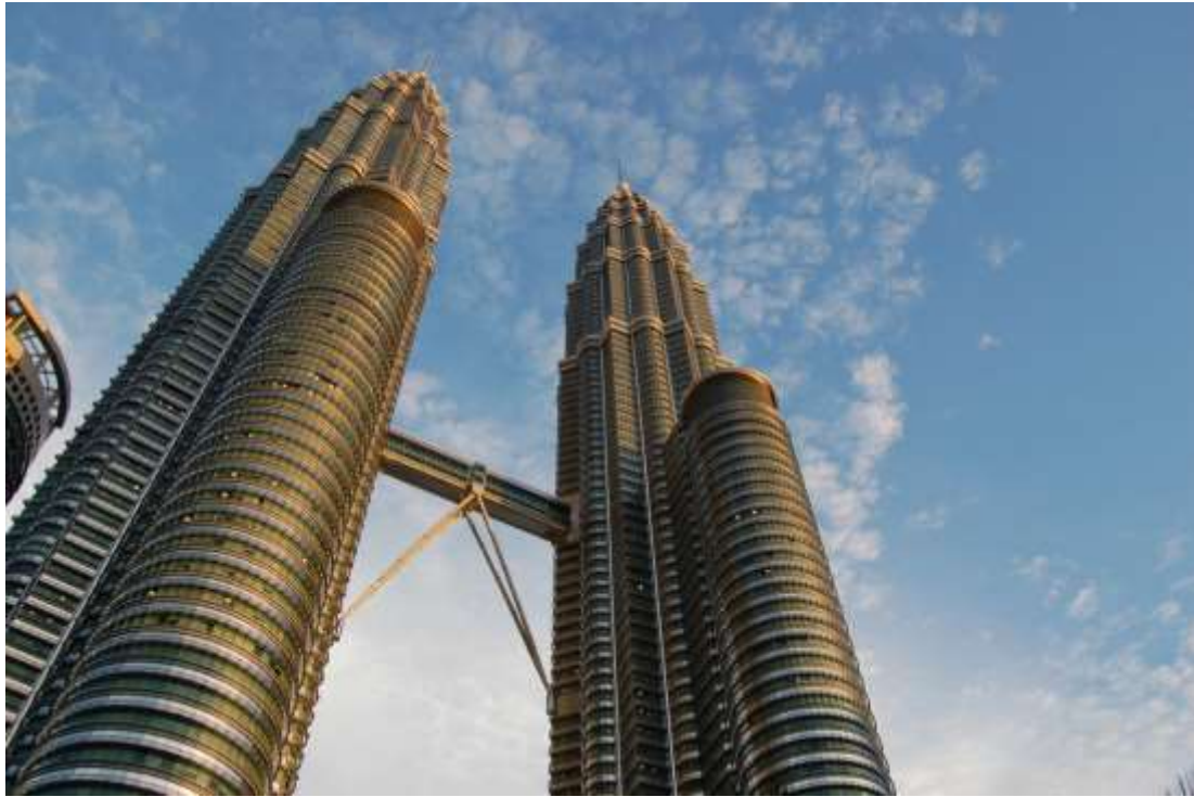
Figure 12. Petronas Twin Towers, Kuala Lumpur, Malaysia, (photo by Luke Watson (Lukeaw_ - Own work).
