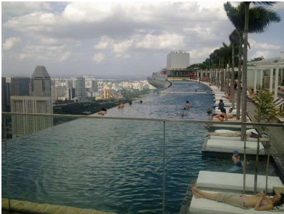
Figure 17. Infinity edge pool on the top of the Marina Bay Hotel, Singapore. (Photo by Walter Lim)
