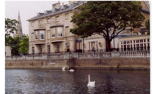
View from the River Ouse, Bedford
