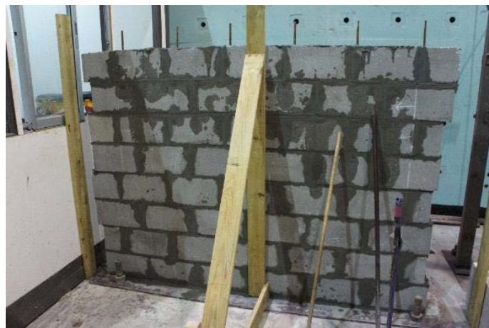
Figure 2: Completed wall test section with regular concrete retaining wall blocks
