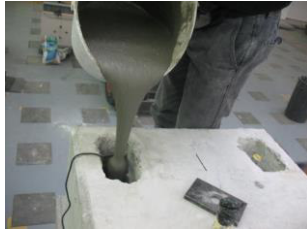
Figure 3. Cast of grout in the beam holes
