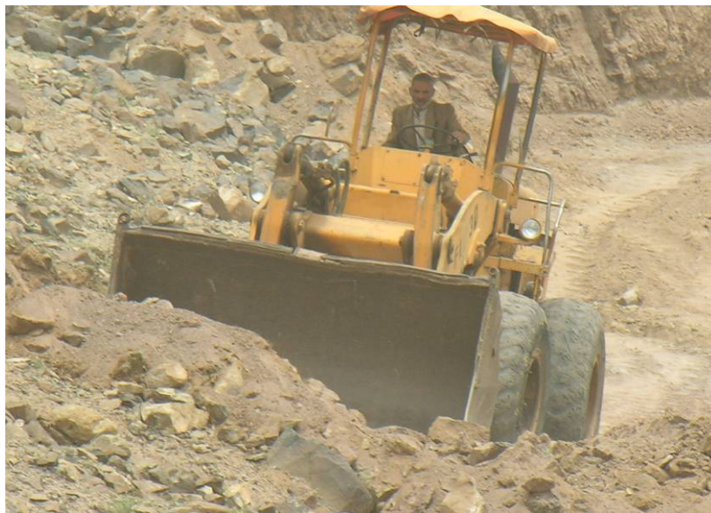
Building new terraces in demined land in Bait 'Oqab
