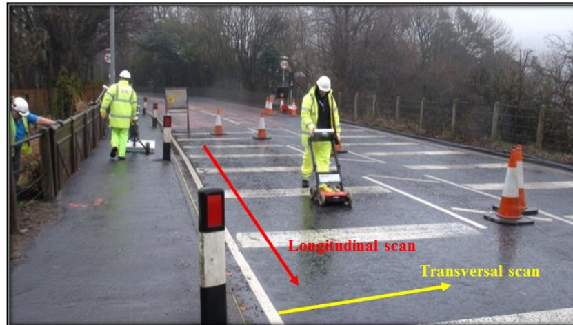
Figure 4.18 – GPR Survey on the west view of the Darvel Road Bridge. (photo taken by Gokhan Kilic, 2010)
