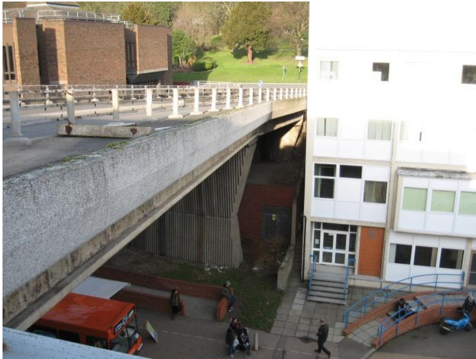
Figure D.19 – South Edge Beam and Parapet
