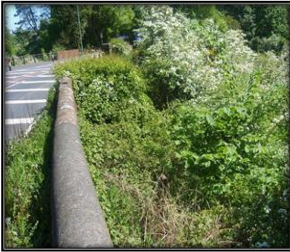
Figure 4.16 – Heavy vegetation North side view of the bridge (photo taken by Gokhan Kilic, 2010)
