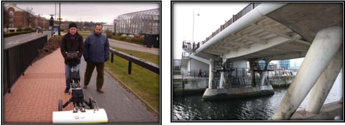
Figure 4.11 – GPR Survey on the St Marys Island Lifting Bridge. (photo from Gokhan Kilic, 2010)
