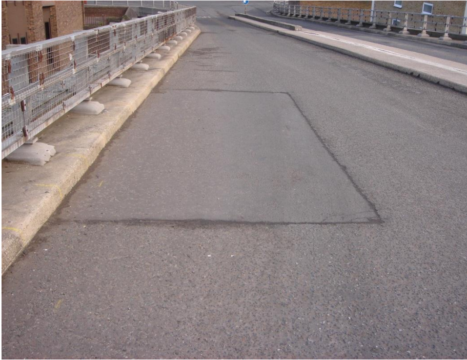
Figure D.21 – Span 1 reinstatement view
