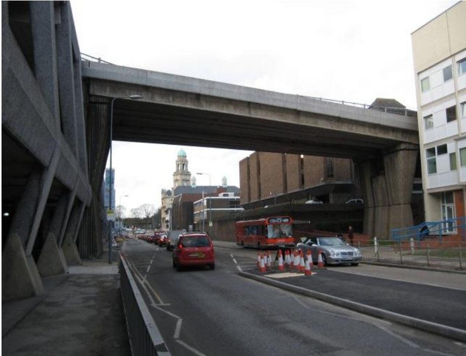
Figure D.15 – South view of Span 1
