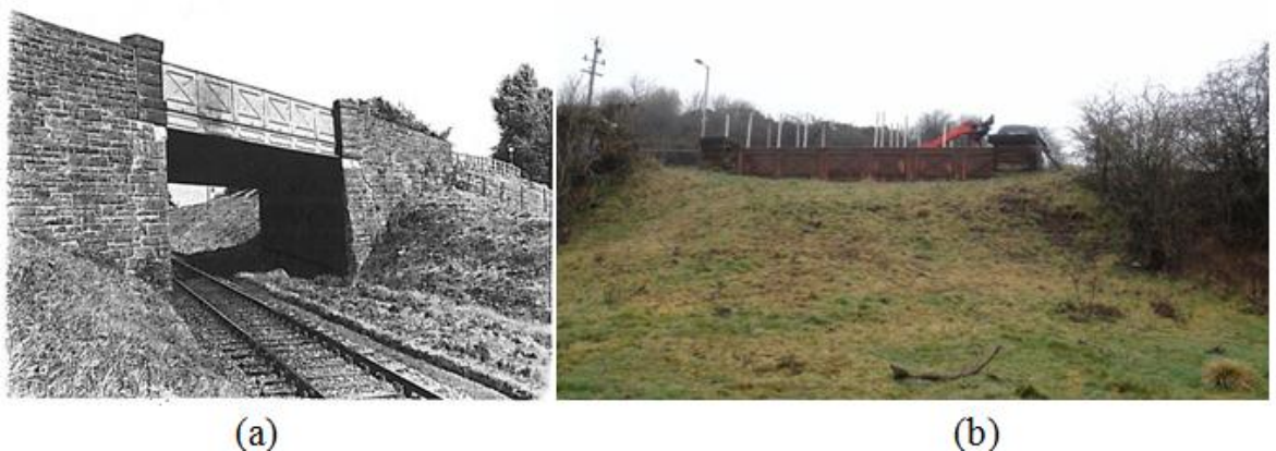
Figure 4.15 – Historic and recent view of the Darvel Road Bridge. (Wikipedia and Picture by Gokhan Kilic, 2010)
