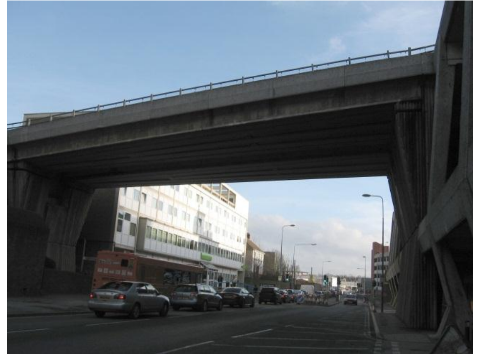
Figure D.16 – North view of Span 1
