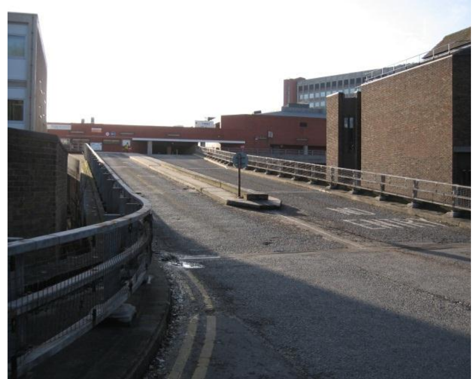
Figure D.18 – East view of structure
