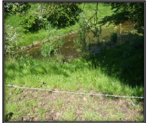
Figure 4.17 – Water ponding on north side of the bridge (photo taken by Gokhan Kilic, 2010)
