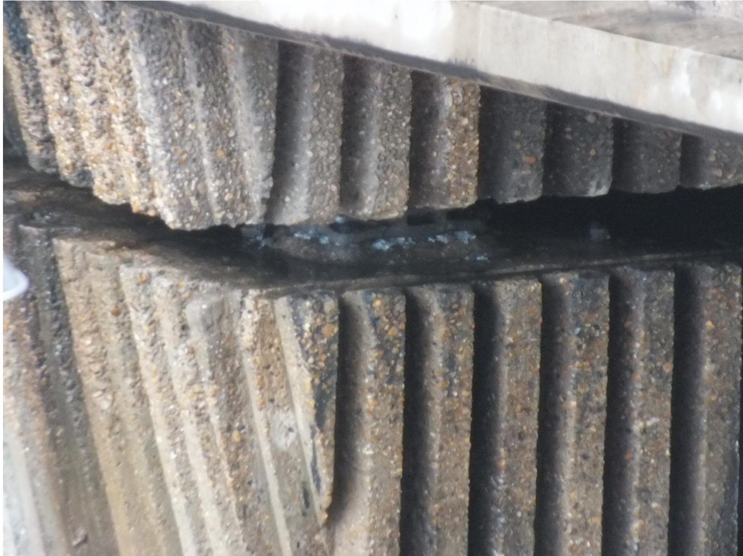
Figure D.5– Pier 2 Bearing
