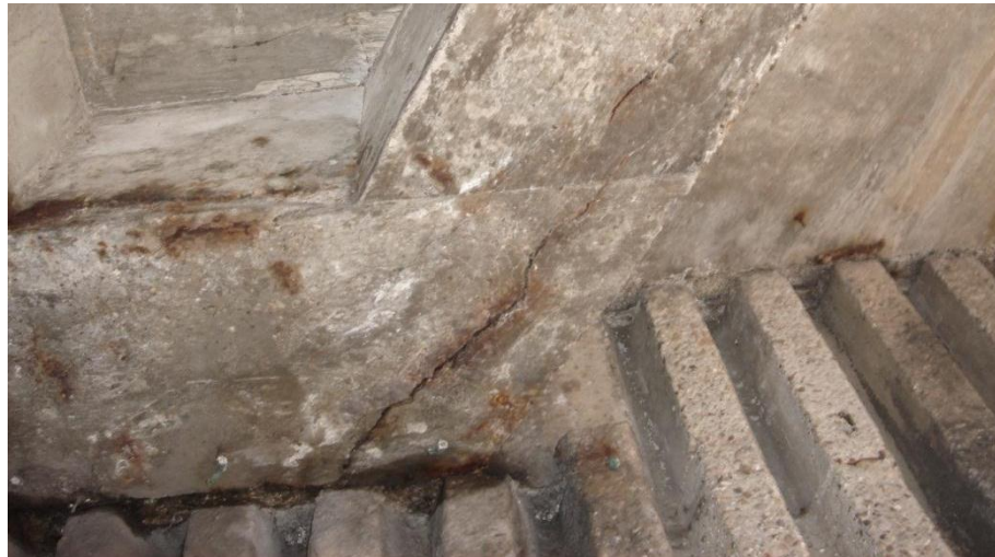
(a) Visual Inspection on 06/07/2010
