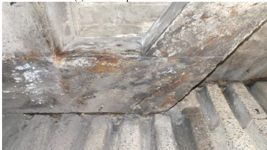
(b) Visual Inspection on 25/06/2011
