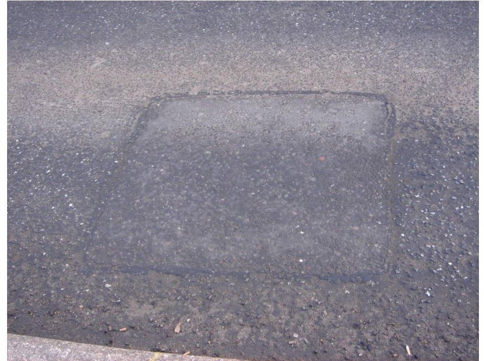
Figure D.22 – Span 4 reinstatement view
