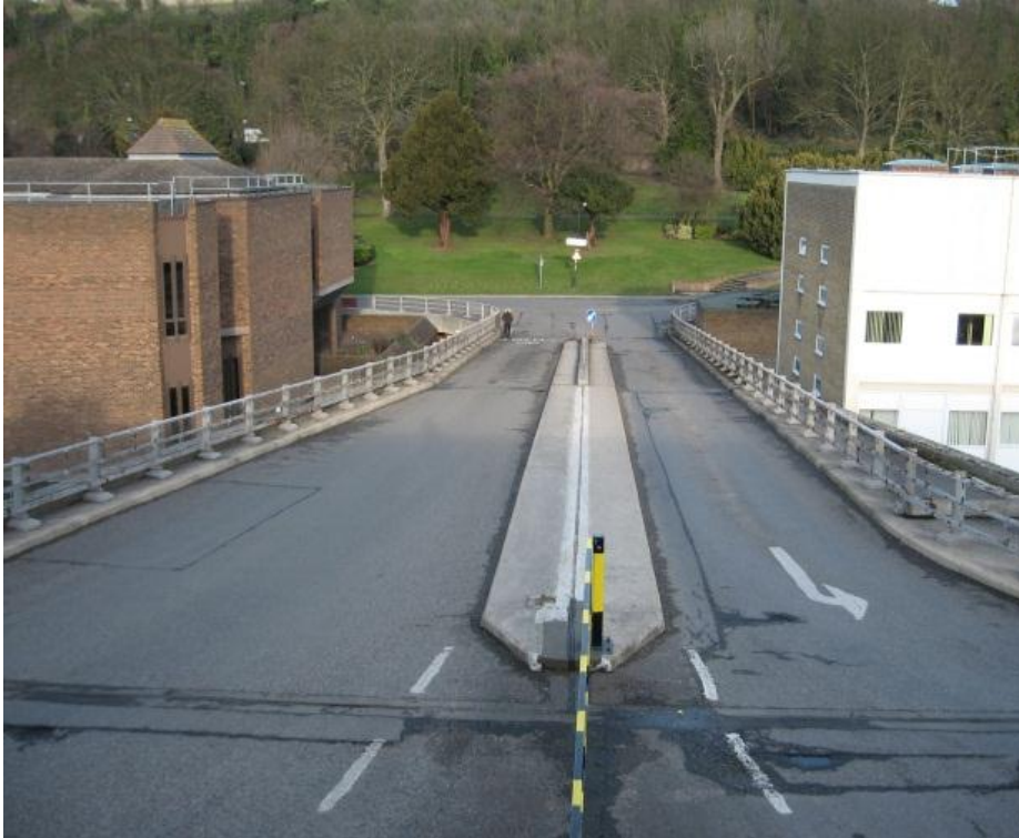
Figure D.17 – West View of structure
