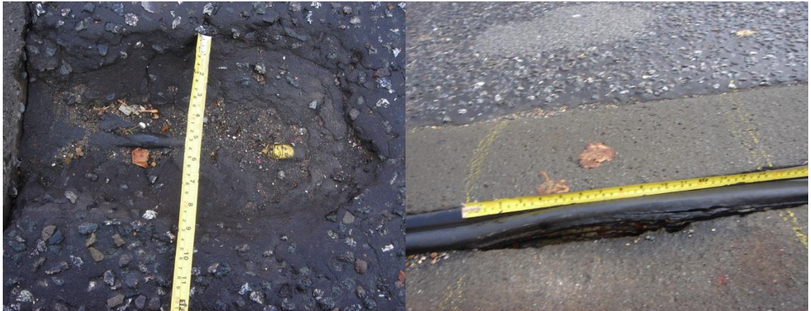
(a) – Asphalt potholes with visible rebar on Span 3 (b) –Expansion joint between span 3 and 4
