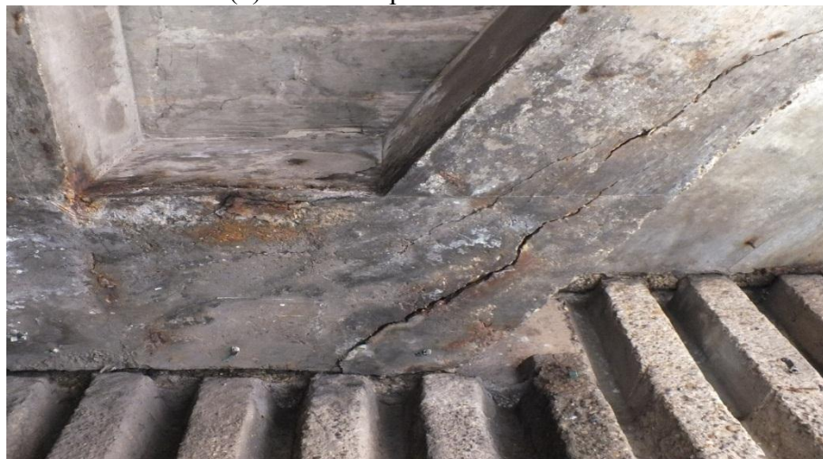
(c) Visual Inspection on 29/07/2012
