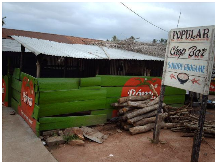
Plate 6.1 A Wooden Chop Bar Building in Sokode
