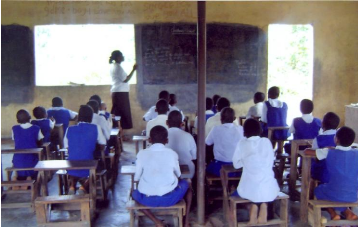
Figure 18: Image showing a classroom of a primary school in Owerri West in need of refurbishment with no doors and windows.
