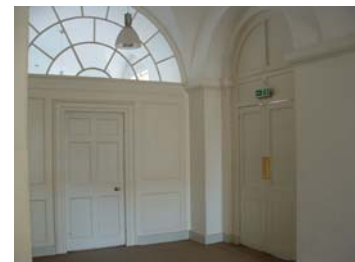
Right view at A12: the front wood exit door on the left and the wood exit door (signed) on the right
