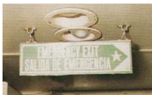
(a) An emergency exit sign installed in the Scandinavian Star [1990]
