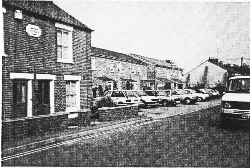
Figure 2.3 Infill development. This illustrates how new build, following selective clearance, can complement an existing area without too much community disruption. The new build properties are set back from the road to allow for parking, a general improvement to accommodate changing needs in older terraced housing stock
