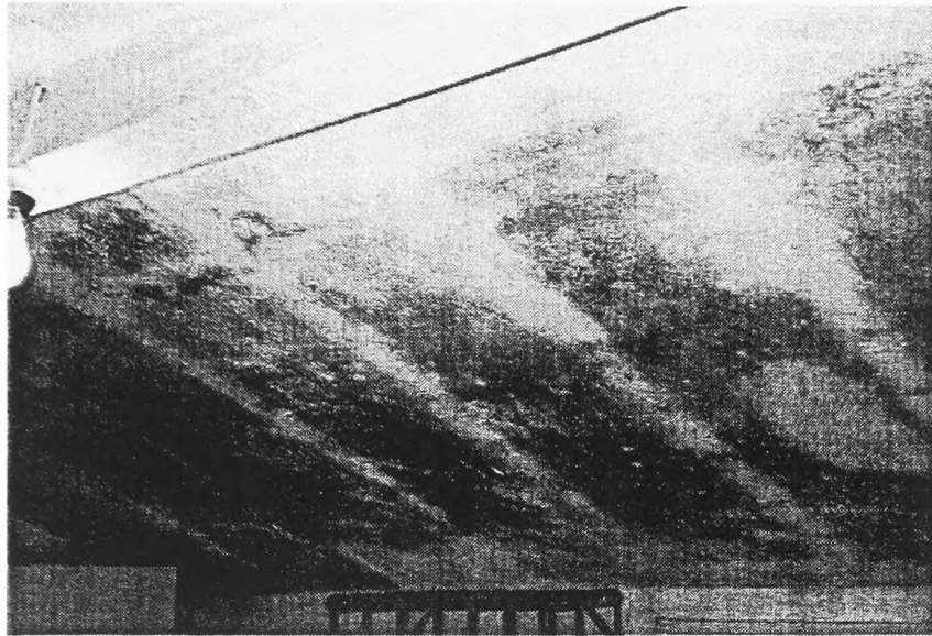
1 2 3 4 5 6 7 8 9 10 11 12 13 14 15 16 17 18 19 20 Figure 2.5 Condensation and mould growth. The condensation and mould growth result 21 from the poor heating supply in the living room as well as inadequate insula- 22 tion and ventilation to this room (the bathroom). The mould growth clearly 23 indicates how it is less likely to proliferate where insulation is provided, and 24 there is no mould growth where the roof joists provide some insulation. In 25 such cases, requiring the landlord to provide an adequate fixed heating source 26 in the main living room and loft insulation, combined with advice to the 27 tenants, would help resolve the situation
