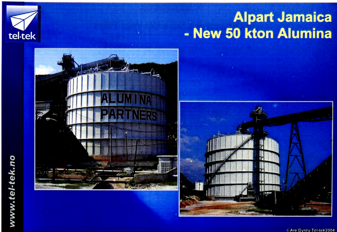
Figure E 7. First sold commercially AS-System at Alpart refinery Jamaica.
