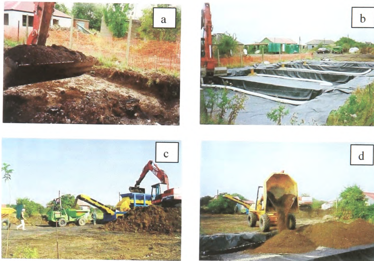
Figure 4.1 – Remediation at Astra Pyrotechnics site (a) excavation of soil, (b) site preparation, lining and drainage construction; (c) soil screening; (d) treated soil backfilling from Blue Circle (2000)
