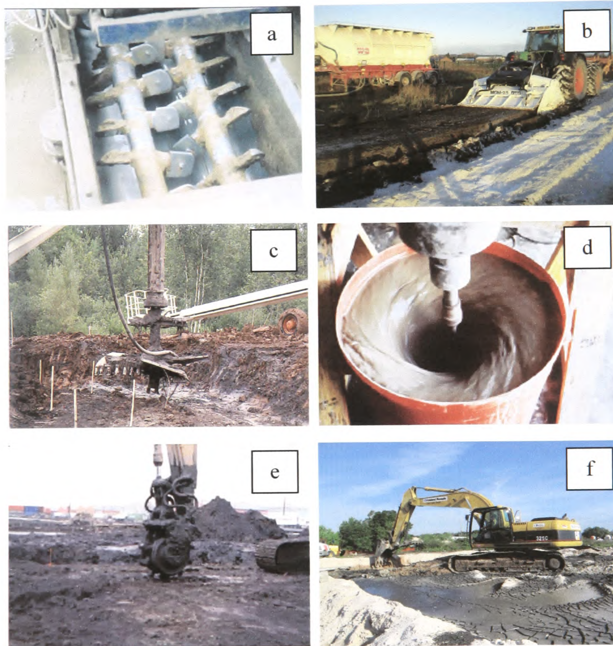
Figure 2.2 – Equipment used for the S/S implementation, in situ and ex situ : a) pug mill; b) rotavator; c) mixing auger; d) in drum mixer; e) in situ blender; f) backhoe
