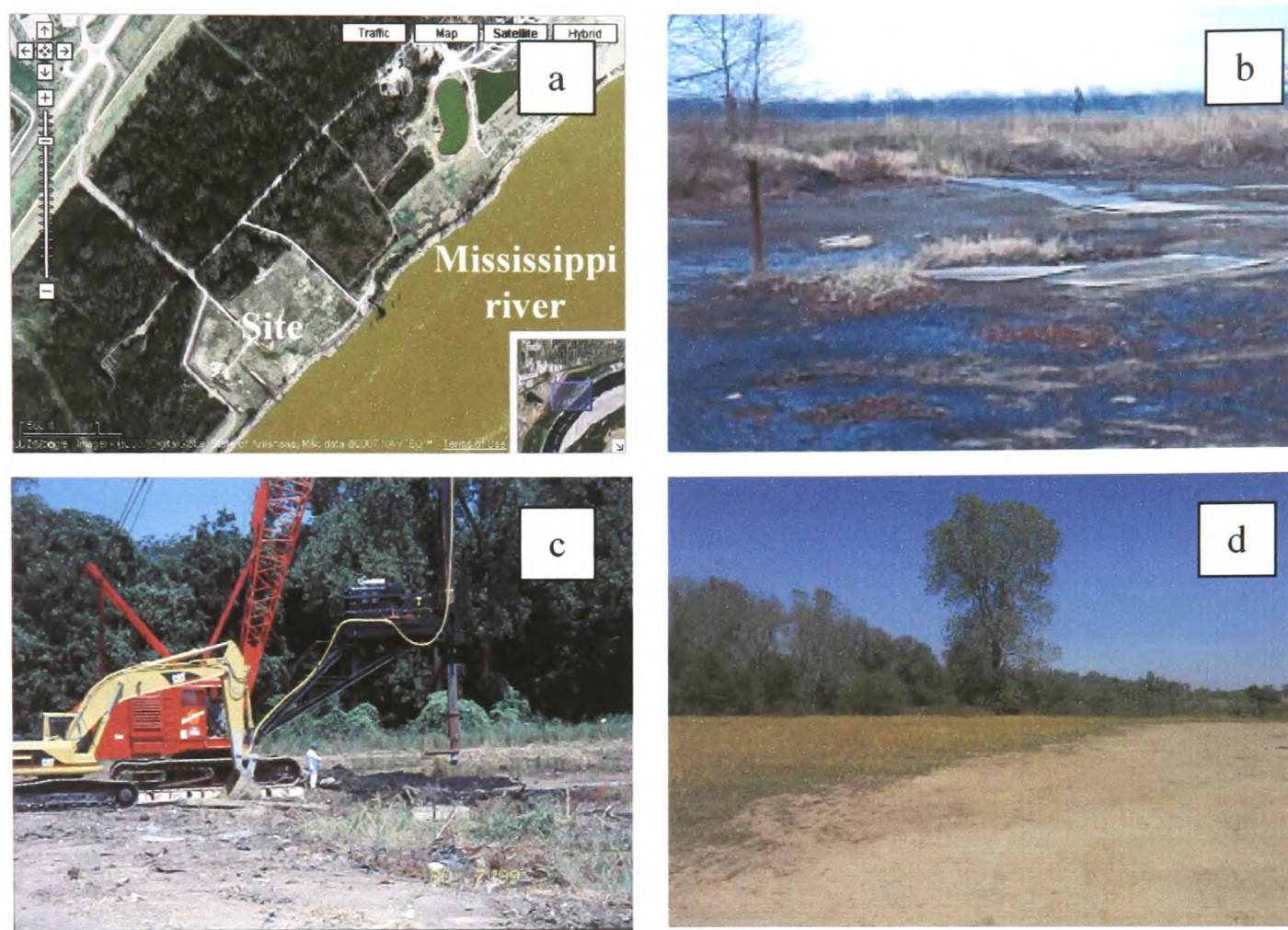
Figure 4.14 – South 8th Street, USA- aerial photograph of the site (a) ( Source: Google Earth TM mapping service; created 17 April 2007 ); the contaminated soils before remediation (b); in situ remediation (c); finished S/S soil (d) (courtesy of Ed Bates)
