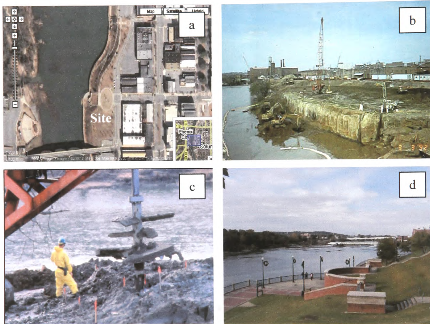
Figure 4.21 – The Columbus MGP site, USA; aerial photograph of the site (a) ( Source: Google Earth™ mapping service; created 17 April 2007 ); site before remediation (b), during and after remediation (c); finished site now a river park (d) (courtesy of Kevin Gardner)
