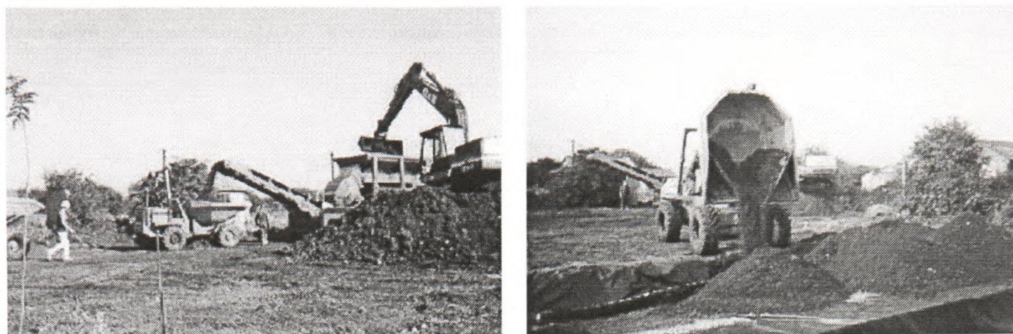
Fig. 1. Soil screening (left) and backfilling in the specially designed cells (right) at the Astra site.
