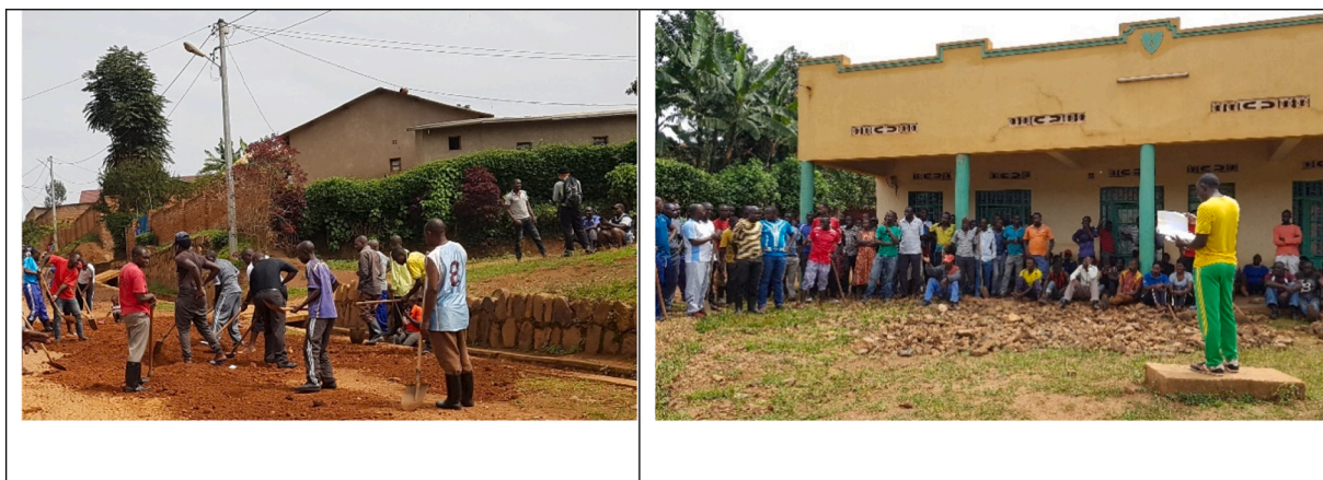
Fig. 5. Public participation in Umuganda in Kigali, 2019. Road repair work as part of the Umuganda in Kigali (left), and Post-activity public meeting (right). Photo credit: Authors.
