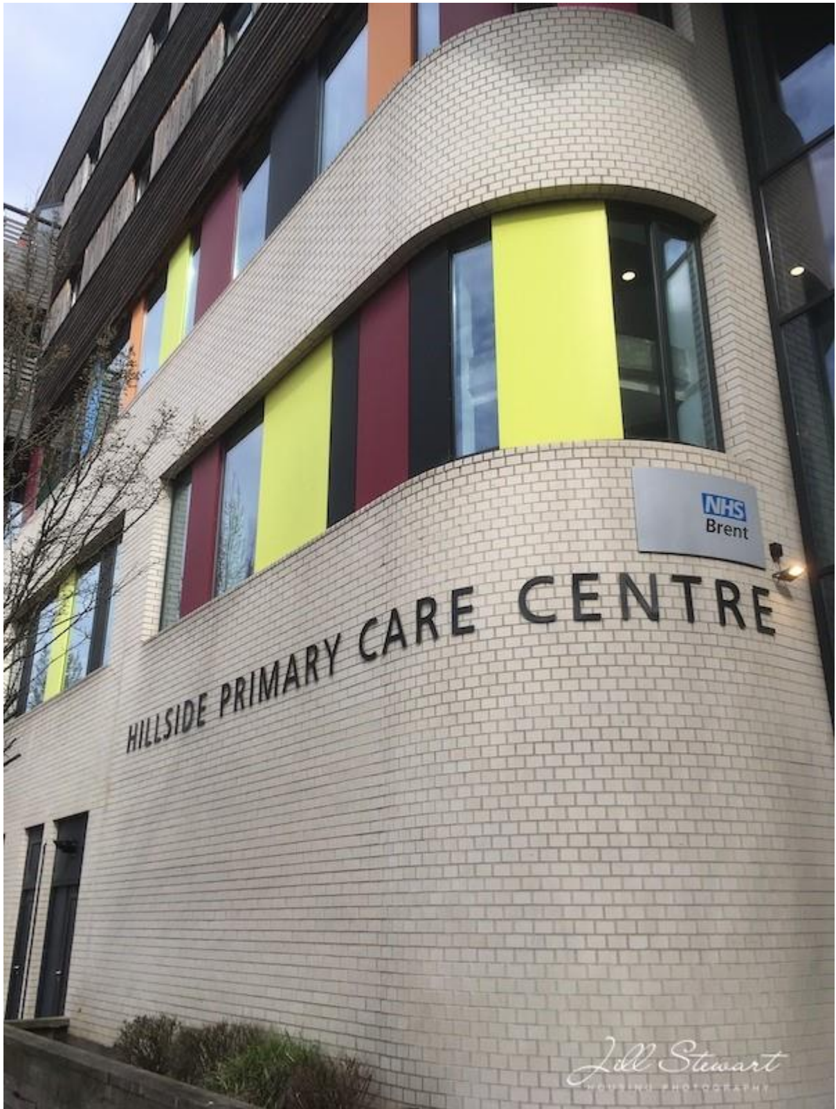
Fig 13: Hillside Primary Care Centre. Photograph ©Jill Stewart, 2023
