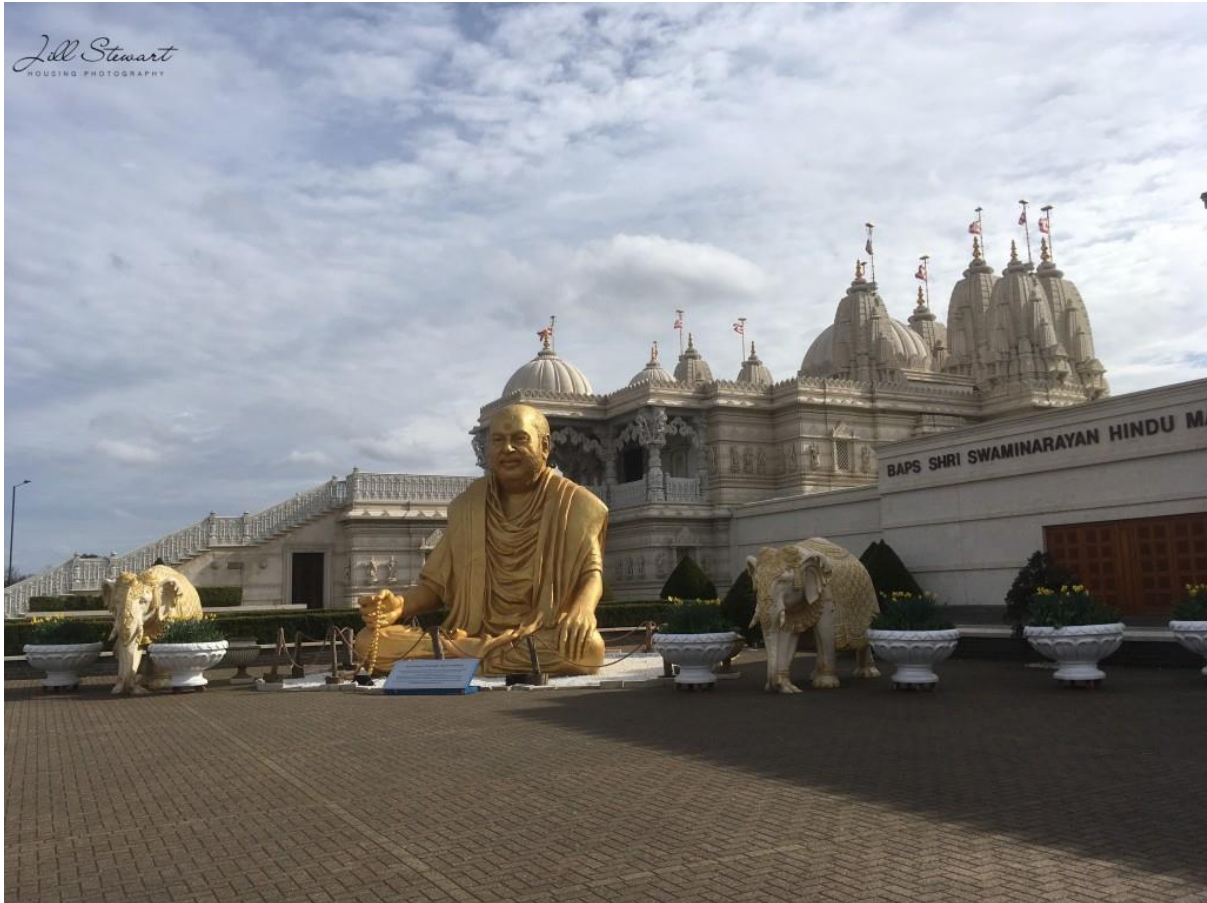
Fig 10: BAPS Shri Swaminarayan Mandir, completed 1995. Photograph ©Jill Stewart, 2023
