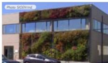
Indirect green facade, Ardoorie (BE)
