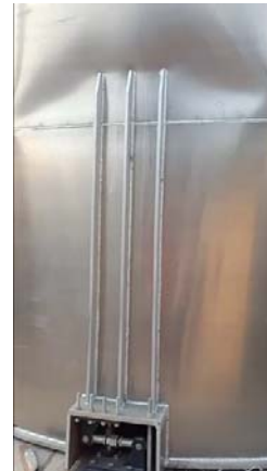
Figure 17 Aluminium silo on load cells, with buckle above stiffeners
