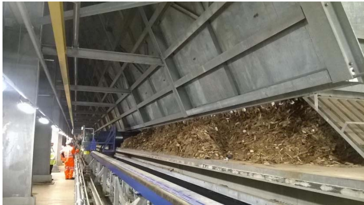
Figure 3 A Large Wedge-Shaped Linear Silo
