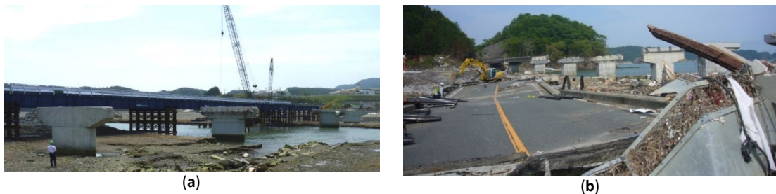
Fig. 1. Damaged bridges after the 2011 Great East Japan Earthquake: (a) Koizumi bridge and (b) Utatsu Bridge
