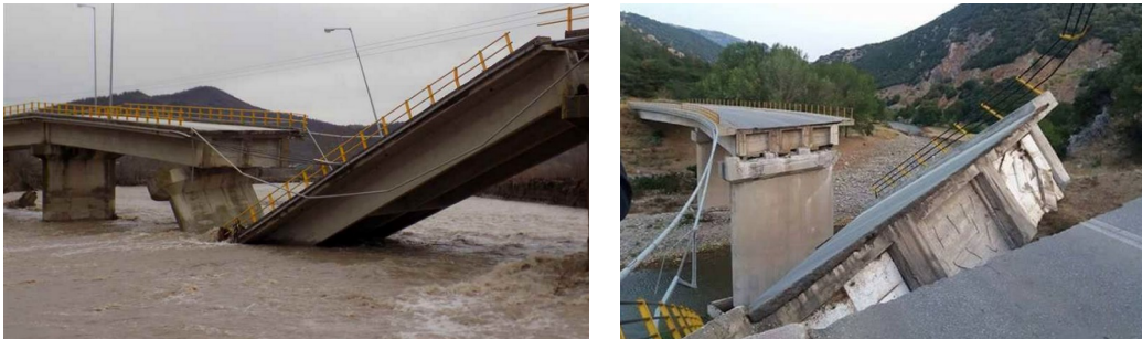
Figure 2: Bridge collapse in Greece (2016-2017) due to flood (left-Kalampaka, Trikala, 2016) and ground movement/foundation slip (right – Iasmos, Rodopi, 2017)
