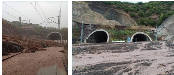
Figure 3. Blockage of the south portal of the ‘Othrios’ twin tunnel, caused by rainfall-induced landslides
