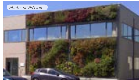
Indirect green facade, Ardoorie (BE)
