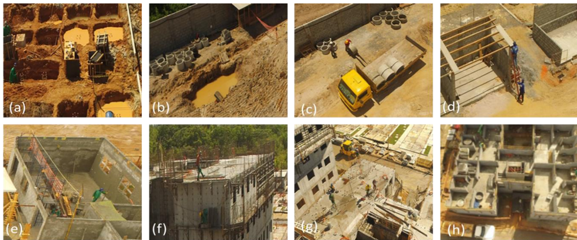
Figure 6: Situations that exceed the safe work limit recorded by UASs during the safety monitoring
