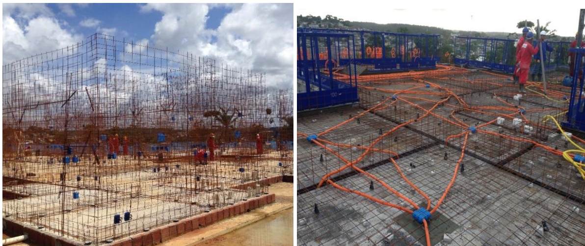
Figure 1: (a) Armature assembly - walls (b) Armature assembly – slab
