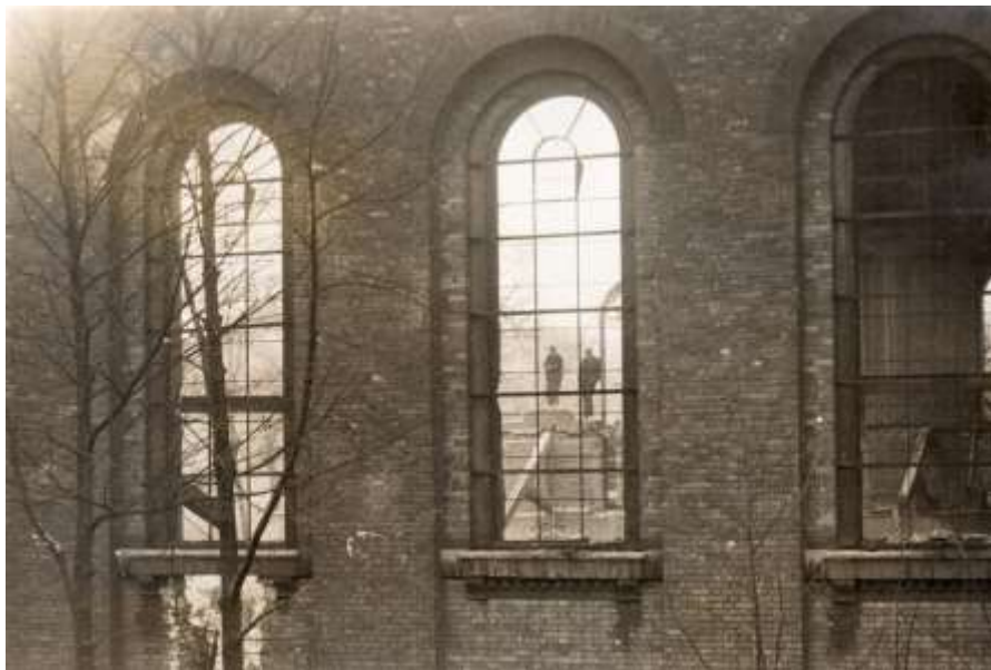
Figure 15. St Mary's Church 1824, Greenwich, George Basevi, south elevation under demolition in 1936. [RGHT]
