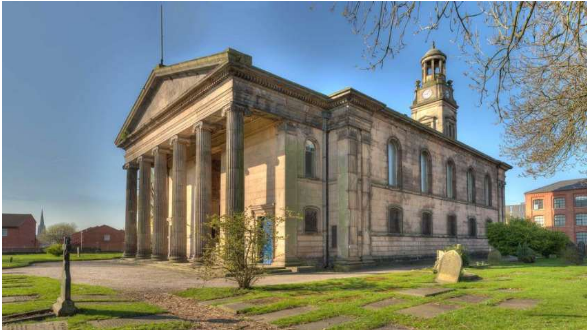
Figure 16. St Thomas' Church, Stockport, northeast view.
