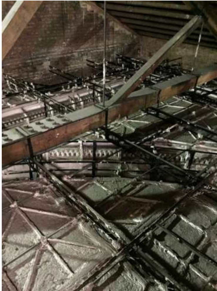
Figure 38. St Alfege Church roof space; view showing the roof structure and the suspended frame supporting the decorative plaster ceiling. [AF June 2017]
