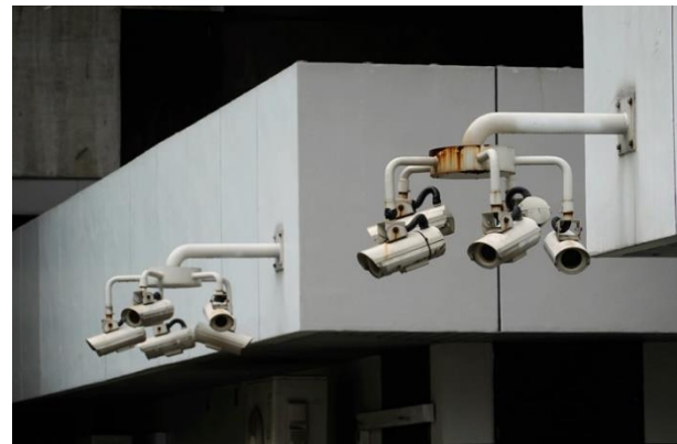
Figure 1: Arrangement of CCTV cameras along Singapore's MRT line
