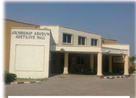
Figure 4: The deep veranda of the hall Source: Researcher's field survey, 2012
