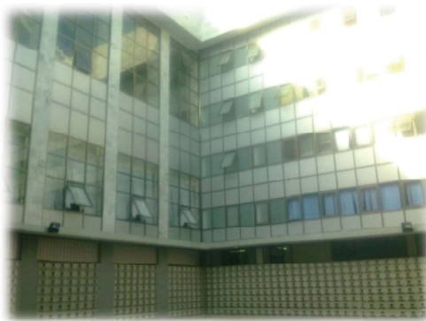
Figure 6: Use of courtyard in the hall Source: Researcher's field survey, 2012
