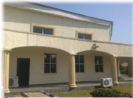
Figure 3: The air-conditioning unit of the hall Source: Researcher's field survey, 2012
