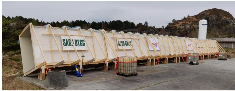
Fig. 2: The Haugesund test facility heeled at 20°
