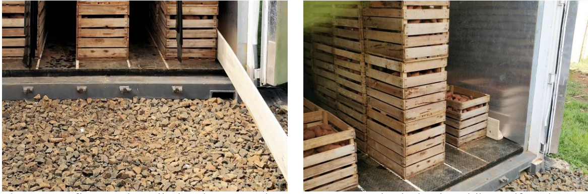
Figure 8 Deflectors installed to improve air temperature and relative humidity uniformity.
