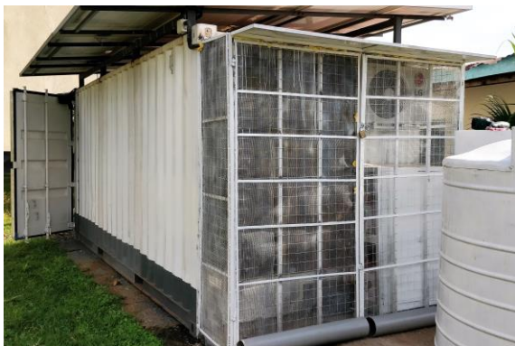
Figure 3 Installation of physical barriers, repellent and traps to protect electrical installation.
