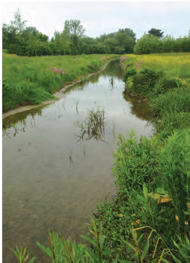
Figure 7.13. This shallow ditch, created as part of a sustainable urban drainage system in Milton Keynes, does not support mosquitoes. It has little emergent and floating vegetation to support mosquito development.
