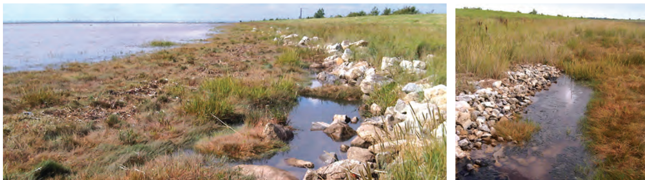
Aedes detritus aquatic habitats on the Humber Estuary associated with a subsidiary bank of ballast adjacent to and in front of a new sea wall.
