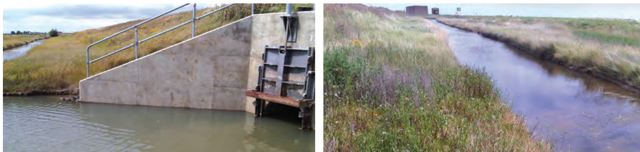
This culvert (left) in Essex was dug to create a new sea wall. The main ditch (right) does not support mosquitoes, but on Spring tides the coastal waters flood the vegetated bank and provide habitat for Aedes detritus larval development.
