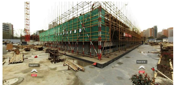
Fig. 4.3 Ground Floor View
