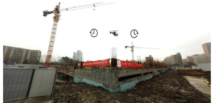
Fig. 4.4. Time Navigation: Early Construction
