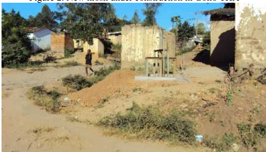
Figure 2. New kiosk under construction in Golio THA
