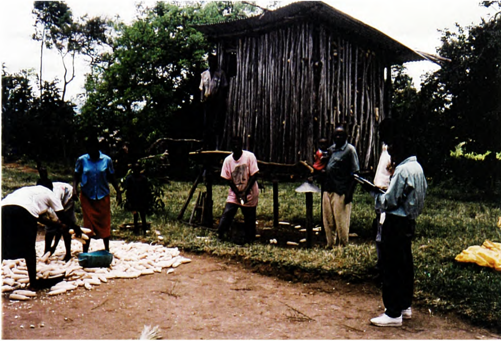
Figure 3.6 . Maize crib built as a demonstration on the farm in Tongaren Division .
