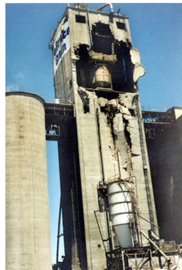
Figure 6. DeBruce Grain Co dust explosion incident [14]
