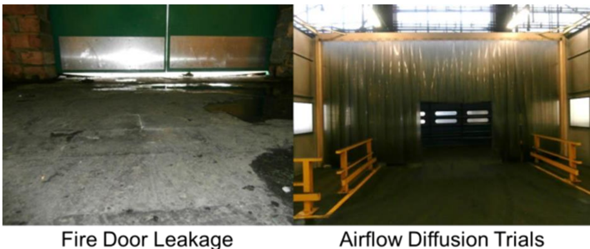
Figure IV: Further leakages at fire doors but also attempts to reduce leakages are shown.
