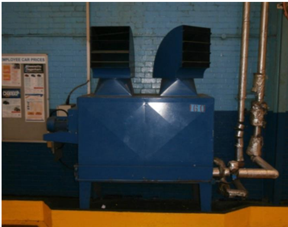
Figure II: Additional heating units which support the main heating system in the DEP. These Units are referred to as "Myson Heaters".
