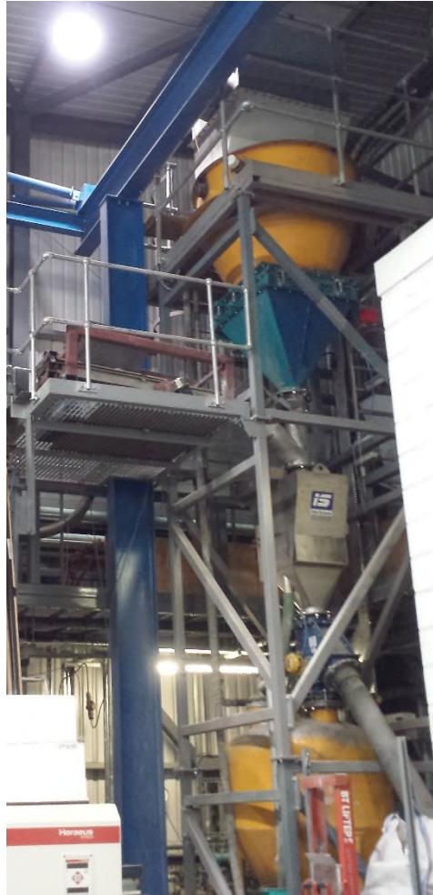
Figure 4-8: Overview of the Pilot Scale Pneumatic Conveying System
