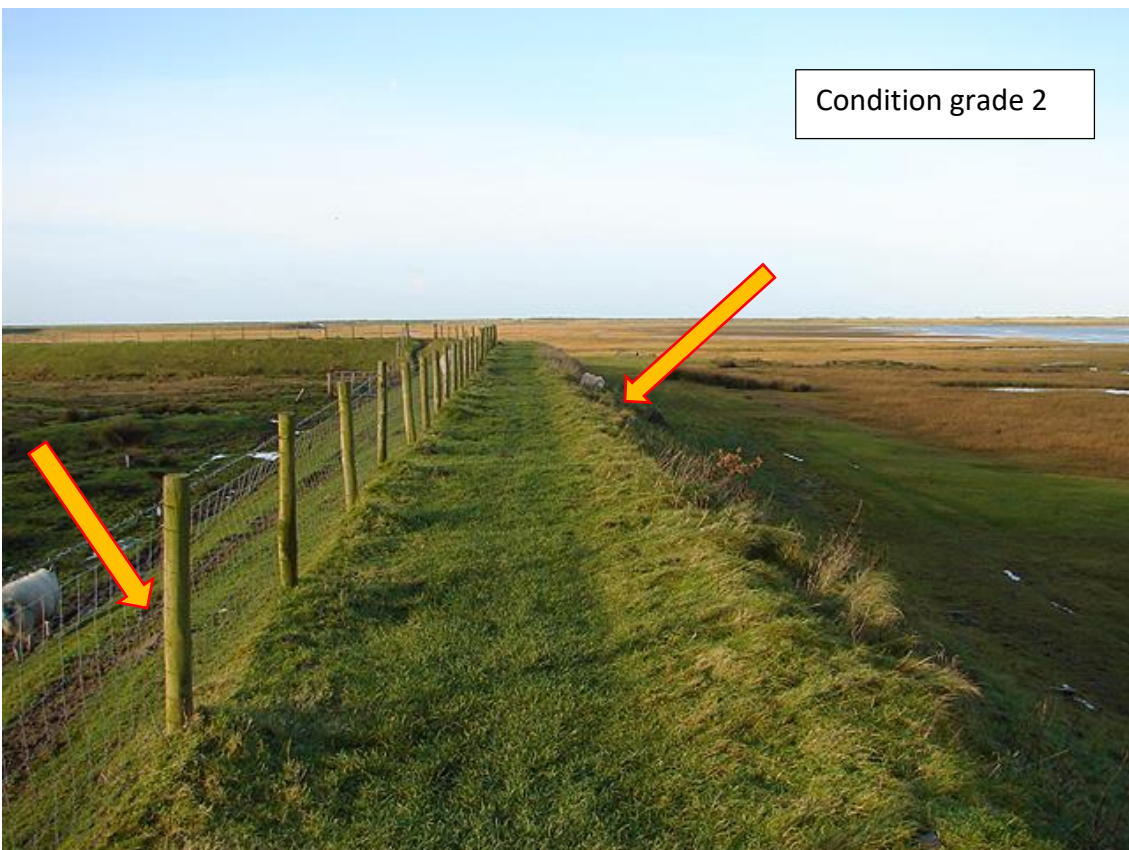
Figure 2.8. Sea defences examples with different condition grades, the second asset is in condition grade 2 due to animal burrow and erosions. The arrows show the defects areas.
