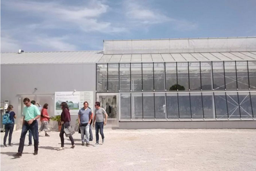
Fig. 21.10 INAPRO aquaponics enclosure with two sections, opaque for fish and greenhouse for plants (Murcia, Spain)
