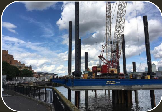
Thames Tideway Tunnel
