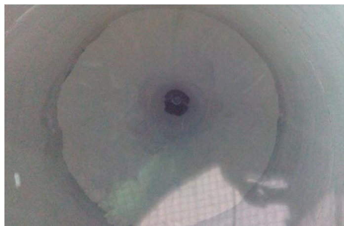
Figure 6.33 Rat-Hole Observed in the Storage Silo
