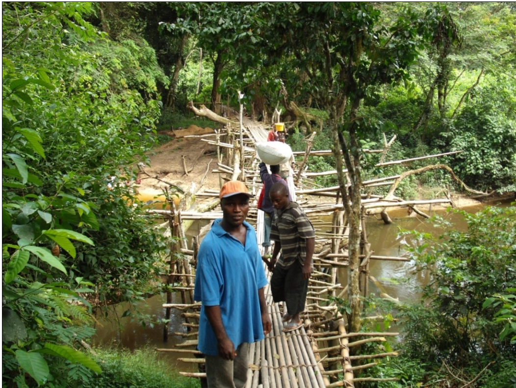
Plate 5.1: Bridge Connecting Barwein Community in Lofa County to Markets
