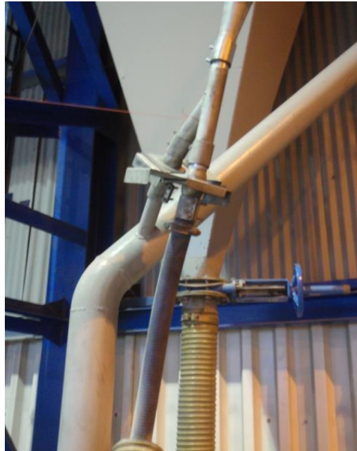
Figure 25 Knife valves on the outlets of the feeding silos for opening & closing alumina & fluoride supply to the feeding air slide and for manual sampling of fluoride.
