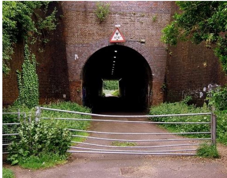
Figure 6.2: Entering the tunnel, moving from light into darkness
