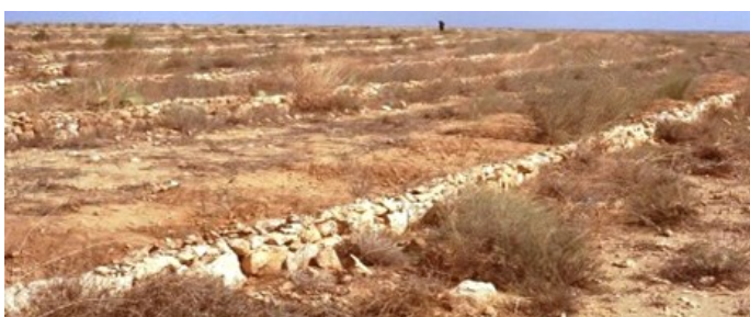
Figure (4): A degraded rangeland in south Tunisia restored with earth works and shrub plantation
