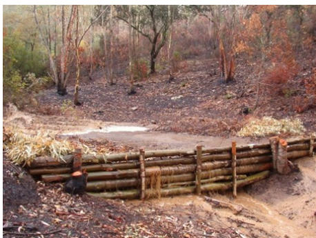
Figure (2): Application of bioengineering techniques for soil and water conservation after forest fires in Cordoba, Spain (Ruiz et al., 2008)
