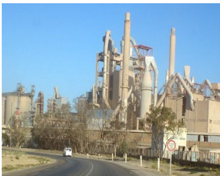
Figure (1): Gabes Cement Plant
