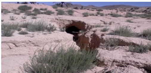
Figure 1: (Above) Degraded land caused by jessour destruction caused by flood water.
