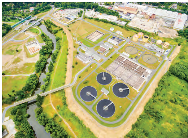
Aerial view of public sewage treatment plant for 165, 000 inhabitants of Pilsen city in Czech Republic, Europe
