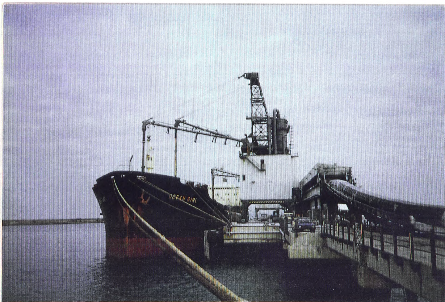
Fig. 2.2 A Present Day Ship Unloader, Holyhead, Anglesey, North-West Wales, Circa 1990.
