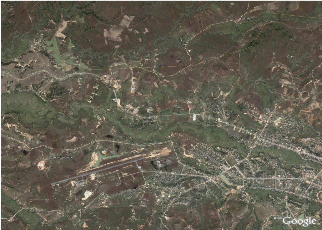
Figure 8. Aerial view of Xieng Khouang runway
