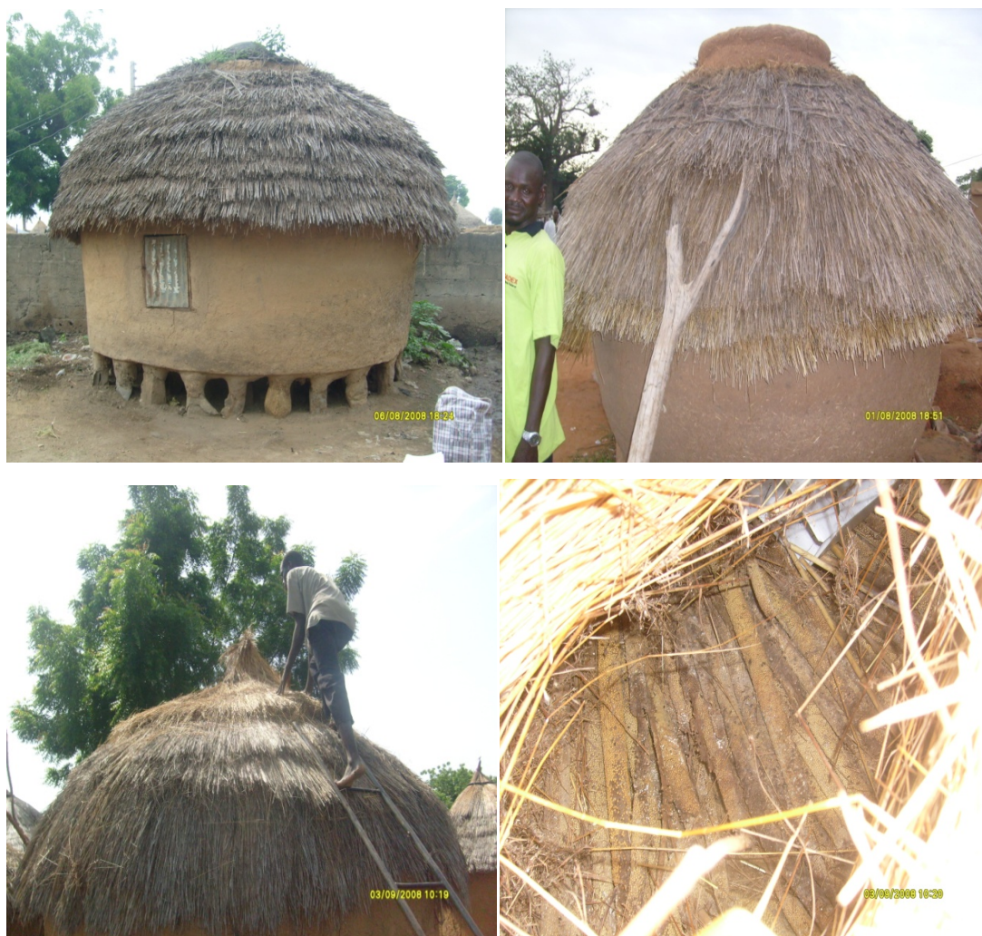
Fig. 4.1 Local granary storage structures (rhombus) in the survey area; window type left top and windowless right top.
