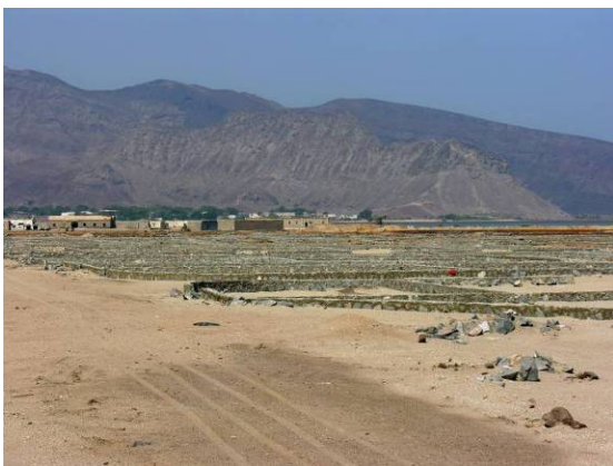
Foundations for 2,600 new houses beside Al-Farsi village
