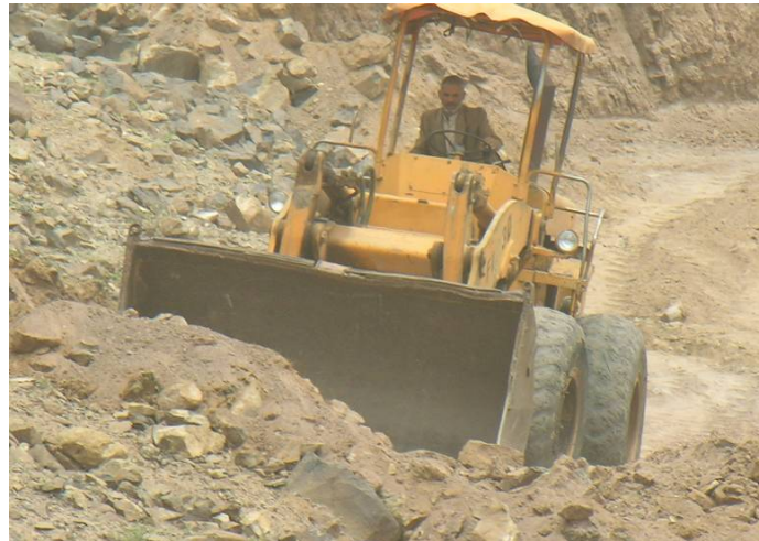
A bulldozer makes new terraces for qat in Bait 'Oqab (Sana'a governorate). At 8000 YR per hour, this method is too expensive for all but the better-off landowners
