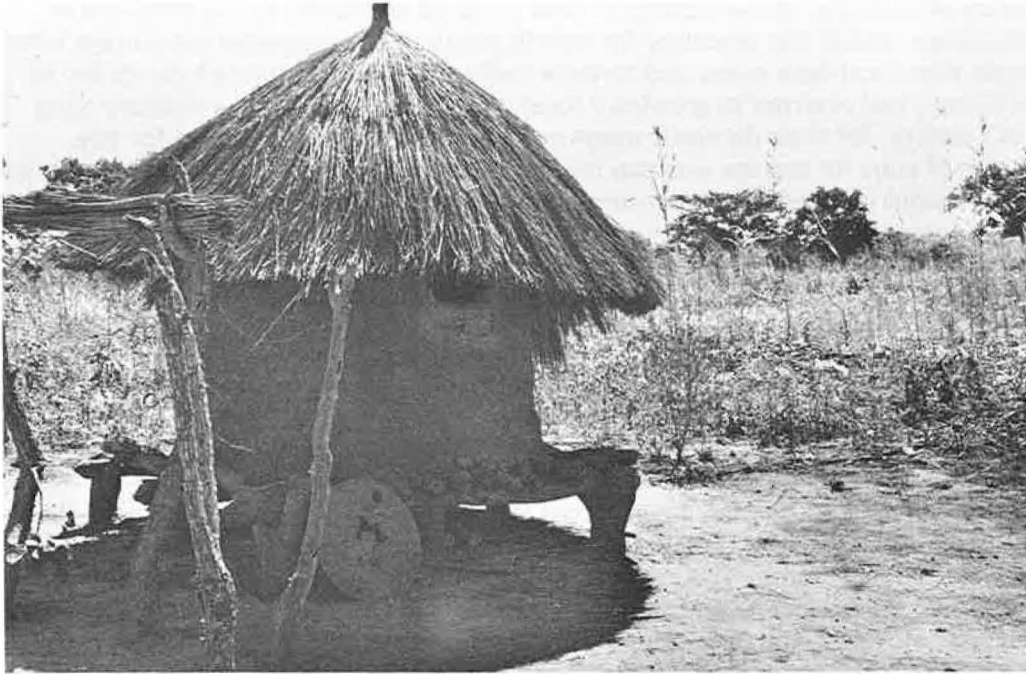
Figure 5 Shelled grain store — muddied internally and externally
