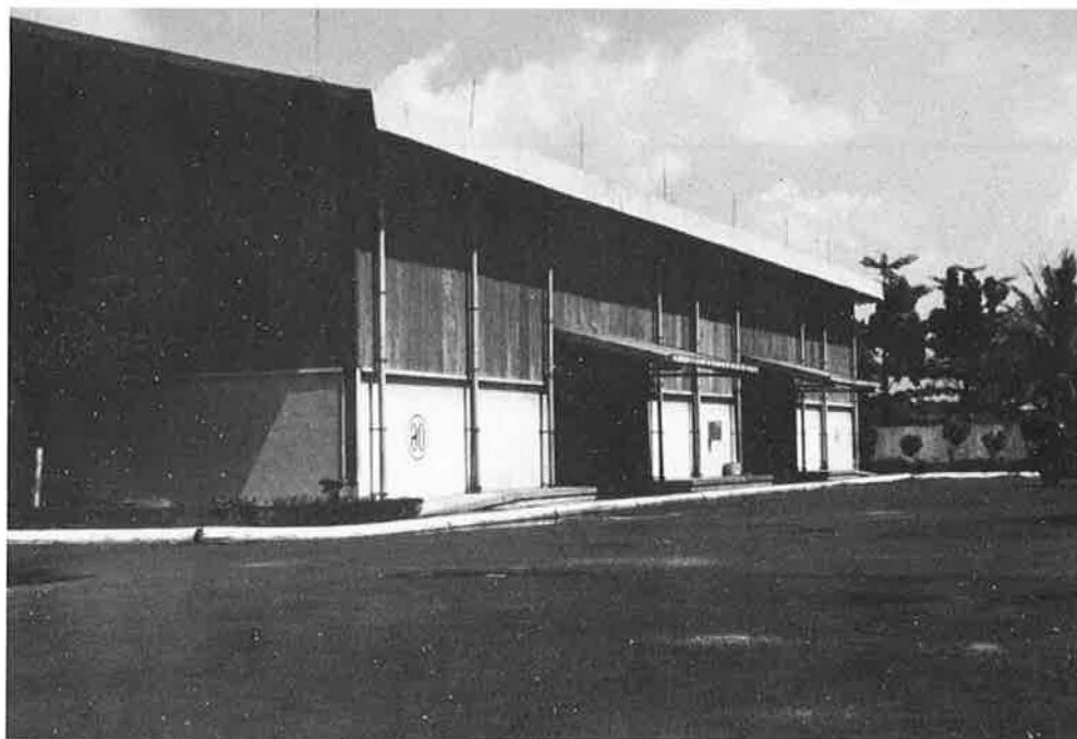
Figure 18 Typical warehouse used for conventional bag storage in the tropics. Under ambient conditions significant changes in grain quality can be predicted.
